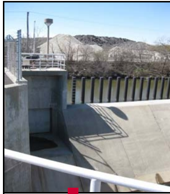
The 7'x7' sluice gate, which diverts flood waters, and the overflow weir.
