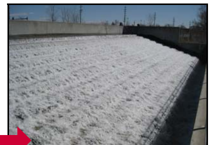
Water flows over aeration facility before returning to Creek.
