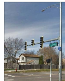
Standard Steel Mast Arm Assembly
