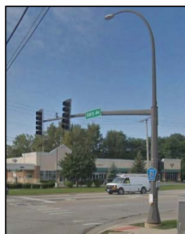
Hexagonal Cross Section Mast Arm
