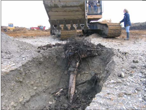
“Mushroom Cap” Fish Crib Installation
