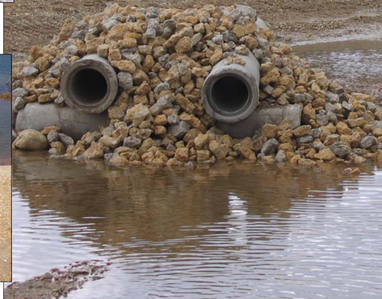
Rock and Culvert Fish Crib at 20ft
